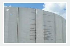
Post-tensioned precast tanks have been a commercially viable alternative to in-situ concrete structures for over 30 years. During this time A-Consult have been at the forefront of product development, being amongst the first to locate the post tensioning tendons within the precast panel and responsible for developing the no maintenance EPDM rubber jointing gasket.
